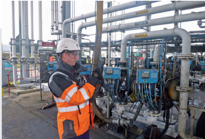
Operation using a portable terminal for a dosage and quantity calculator for loading tank trucks
